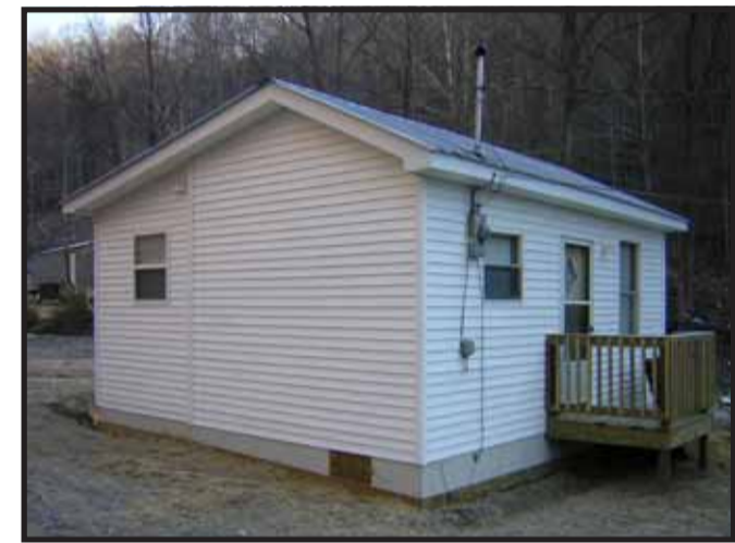
The final product with the housing CORE in place
