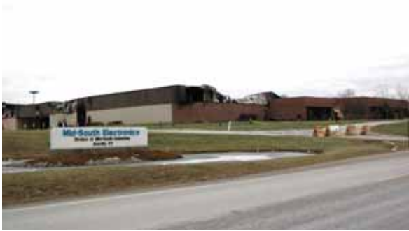
Pictured above is the Midsouth plant after the fire.
