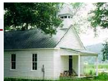
EZ funds saved the Hopkins School in Albany, which was built in the early 1900s but had fallen into disrepair.
