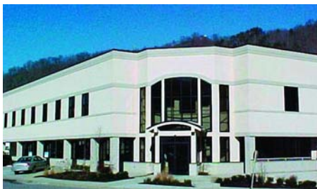
By installing fiber optic cable in rural Kentucky, SouthEast Telephone of Pikeville is helping residents better prepare for a 21st century career and compete in a global economy.
